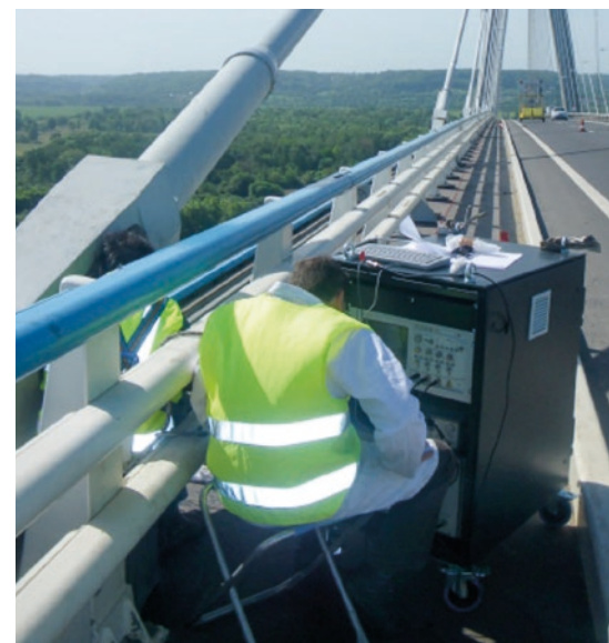
IFSTTAR inspection device in operation on site
