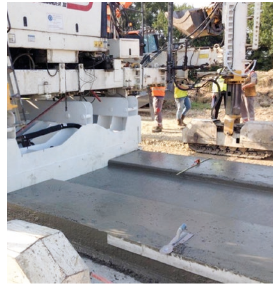
Construction of the rolling track demonstrator using the slipform paver
