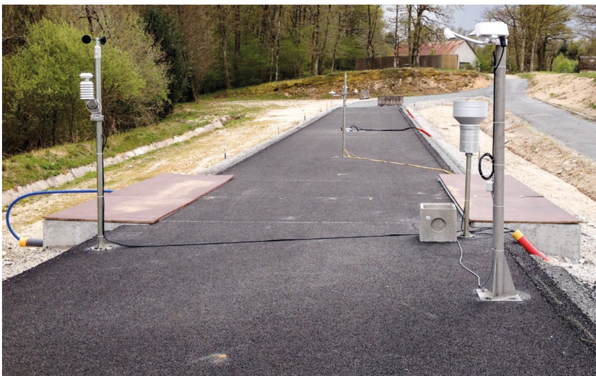
Demonstrator for thermodynamic self-heating roadway in Egletons
